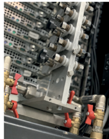
Connecting manifold to Facility Water System
