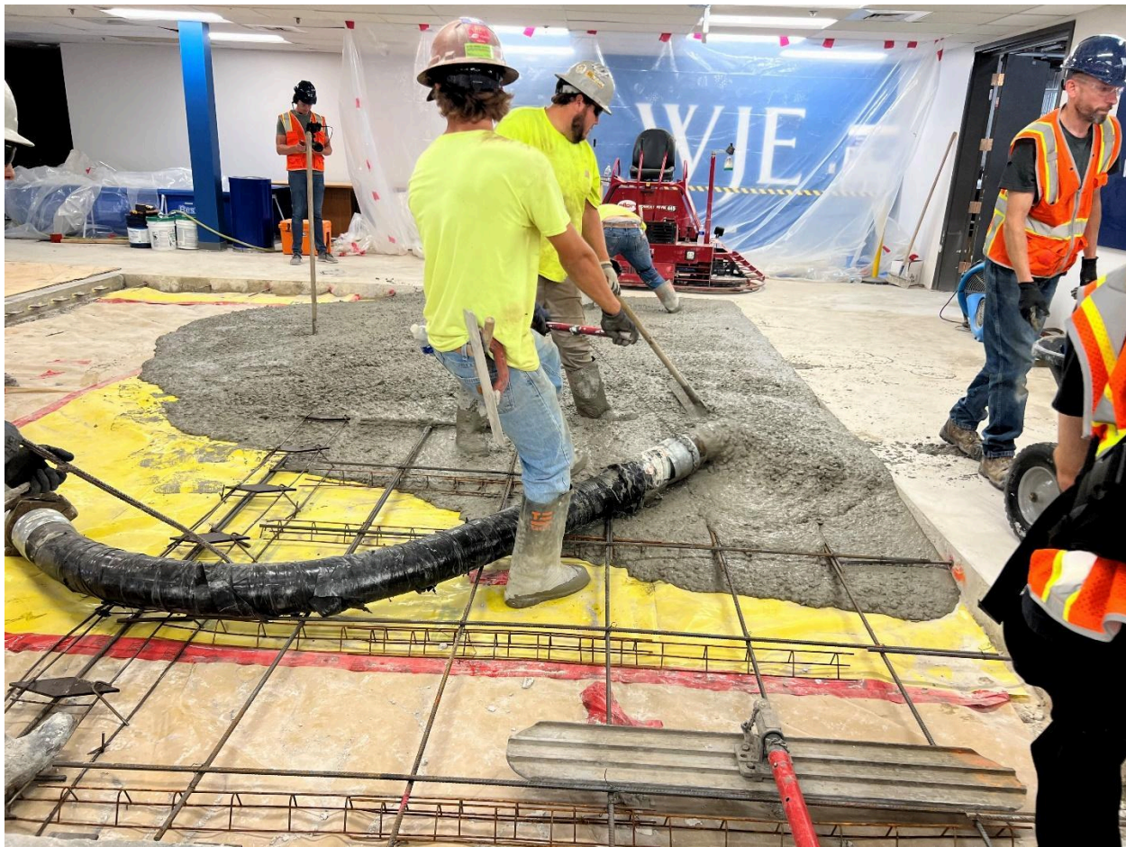
Figure 16. Representative photo of Slab 2 placement with Mix 2.
