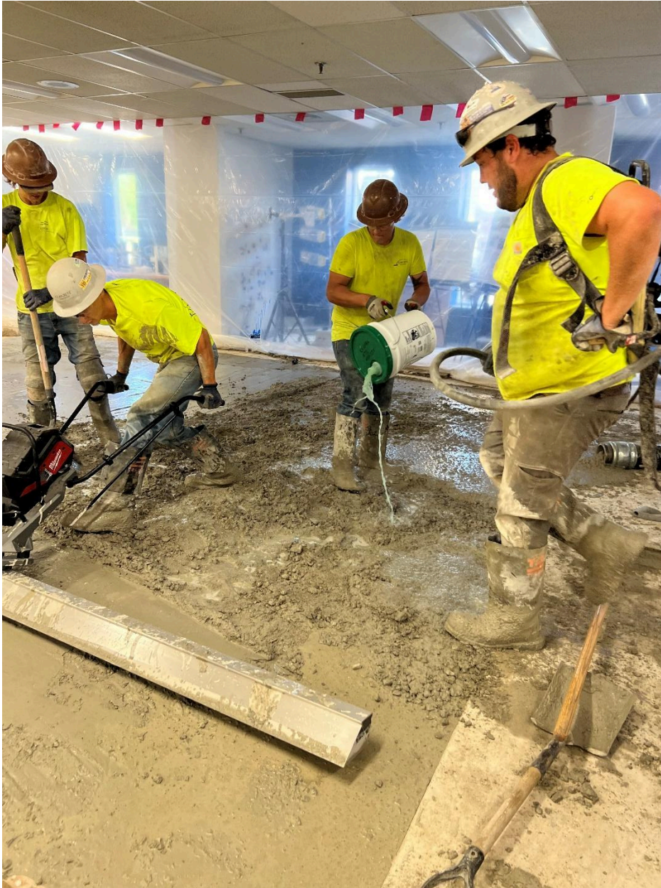
Figure 23. Evaporation retarder application to Mix 3 to facilitate vibratory screeding at Slab 3.
