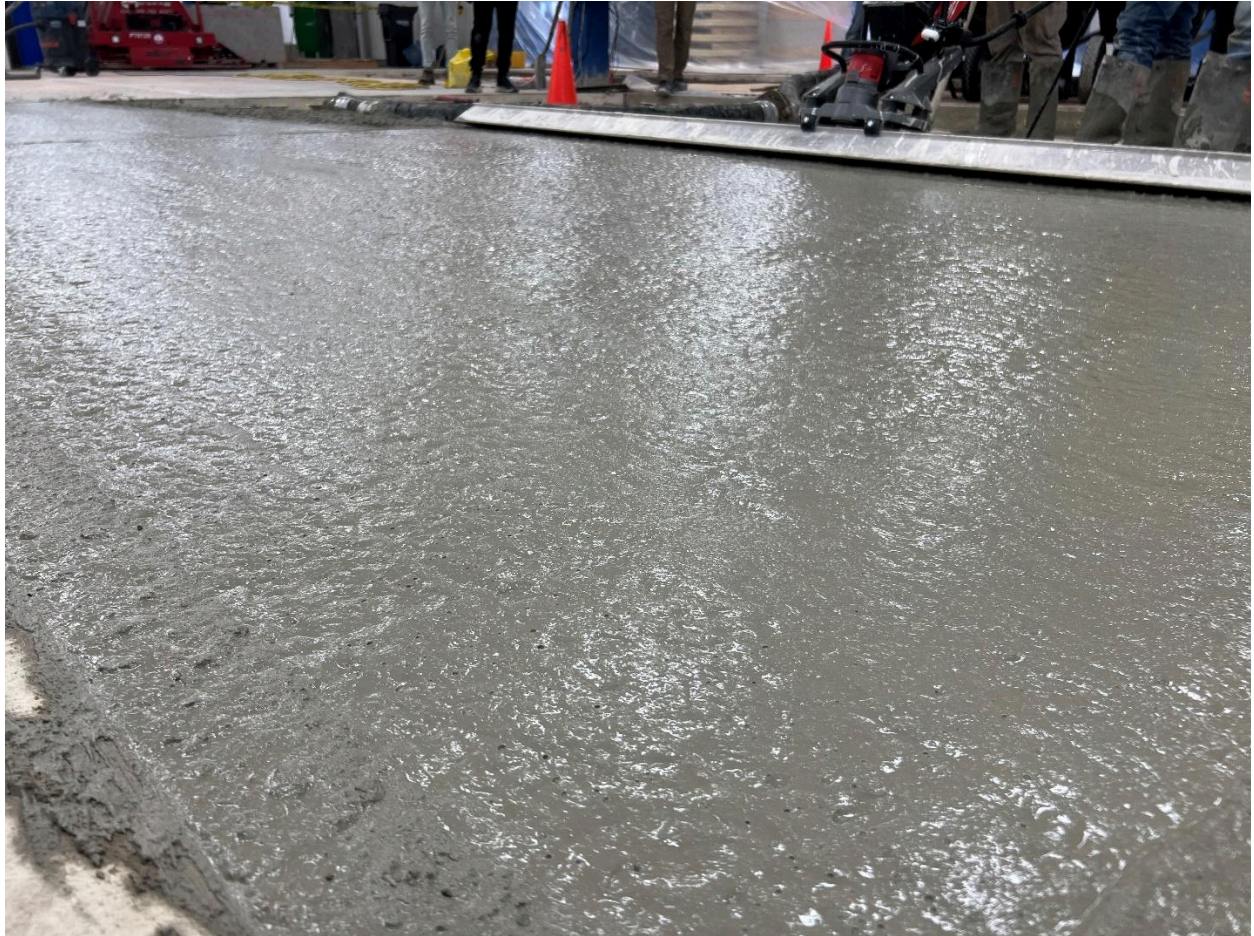
Figure 17. Slab 2 Mix 2 close-up photograph of concrete surface following vibratory screeding.
