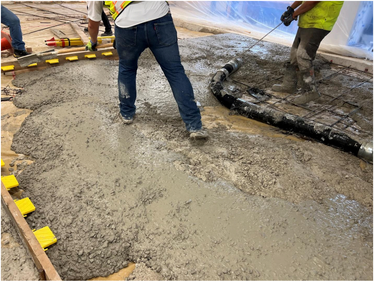
Figure 20. Representative photo of Slab 3 placement with Mix 3 upon initial pumping and placement of Truck 1. Note some aggregate segregation.
