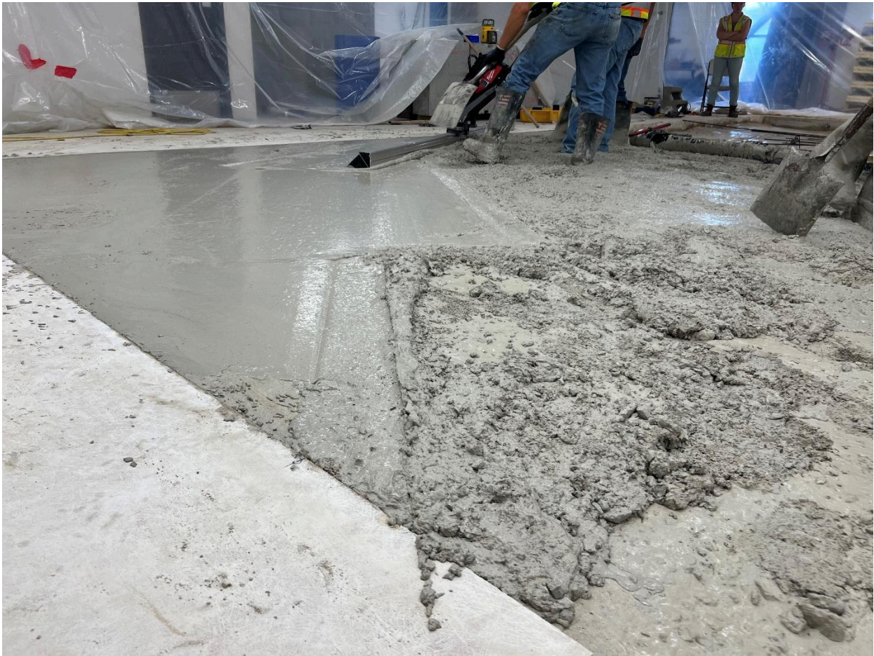
Figure 28. Representative photo of Slab 4, Mix 4 after mix became stiff and more difficult to move.
