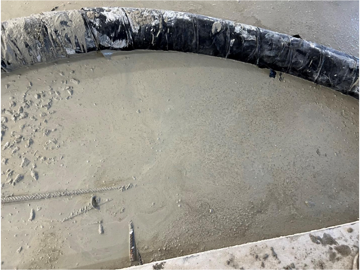
Figure 21. Representative photo of Slab 3 placement with Mix 3 upon initial pumping and placement of Truck 2. Note aggregate and paste segregation.
