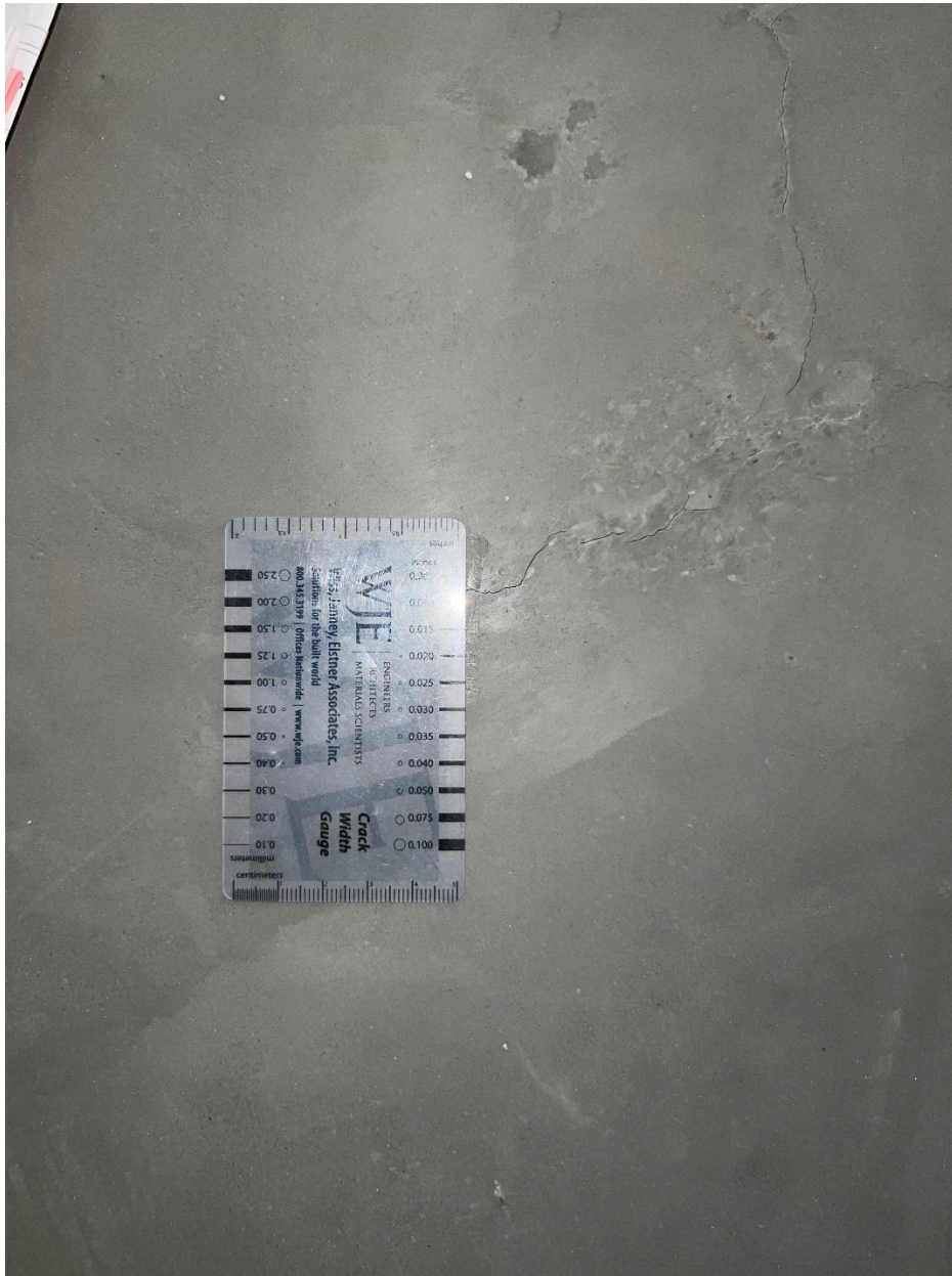
Figure 26. Plastic shrinkage cracking in Slab 3 following completion of power troweling.
