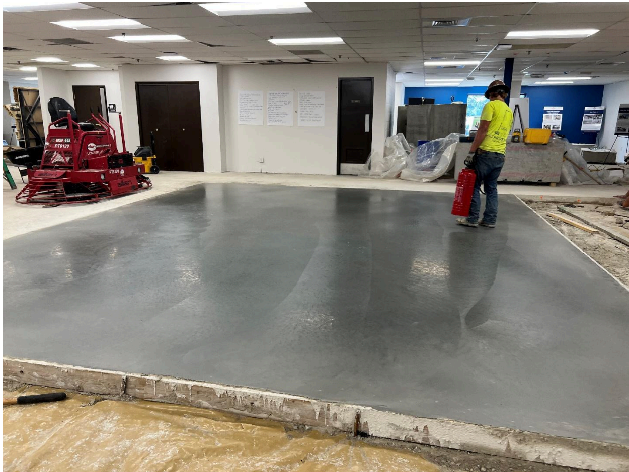
Figure 32. Slab 4, Mix 4 after completion of placement and power finishing. Application of densifier via spray canister commencing in photograph.
