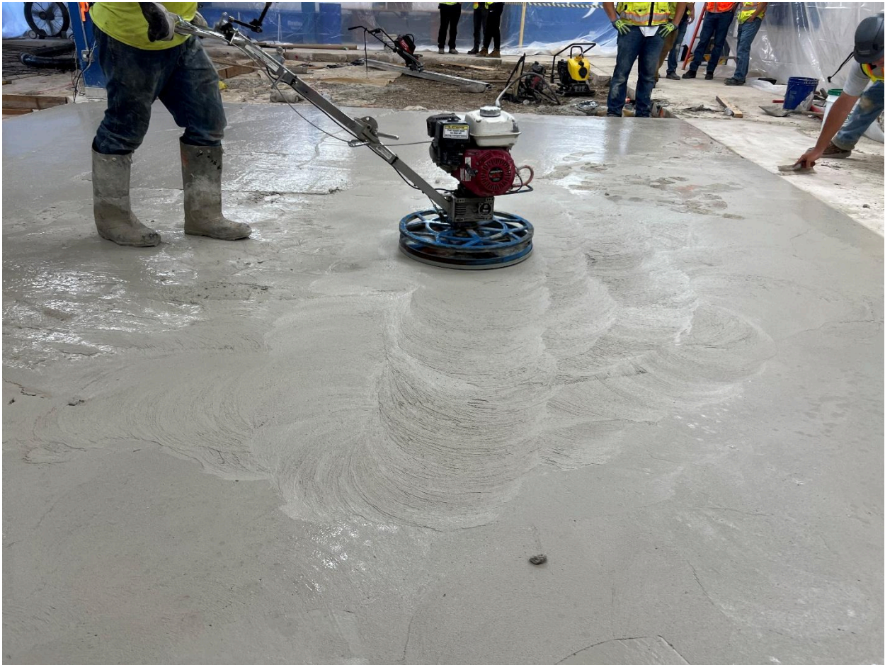
Figure 31. Slab 4, Mix 4 walkable pan finishing at edges.
