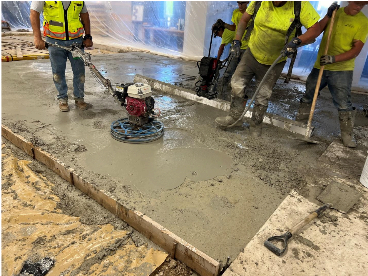
Figure 24. Slab 3 during placement showing use of pushable pan finisher.
