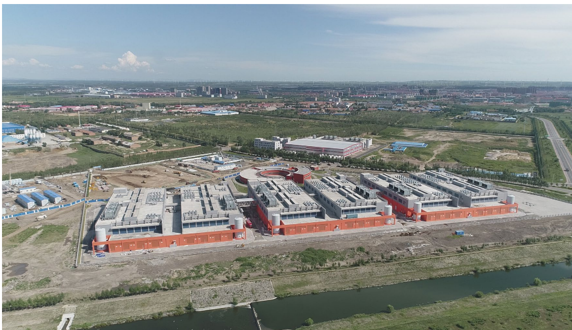
The Alibaba Cloud Zhangbei Data Center - No.1 Campus - Phase II Project was designed and built independently by Alibaba. The vacant land in the figure was the state on August 10, 2018 and the buildings were capped on October 29. Across the road is the Phase I Project. By observing carefully, you can see dense wind turbines at the distant near the skyline
