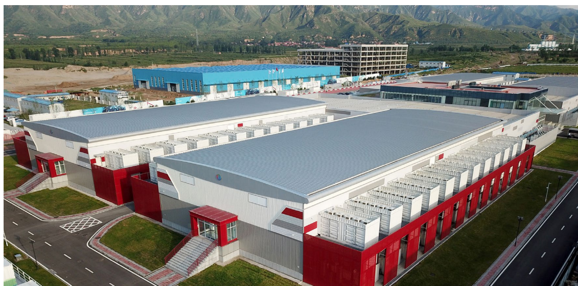
Phase I Project of ByteDance Huailai Data Center: the white building at the foot of the mountain (top right of the picture) is a substation
