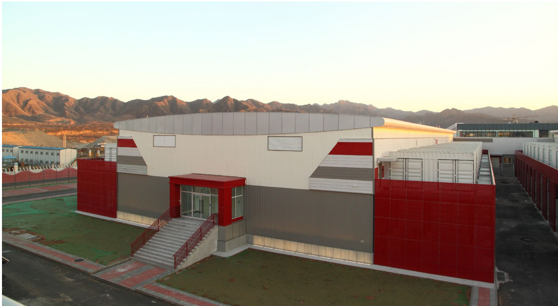
One computer room module in Phase I Project of ByteDance Huailai Data Center
