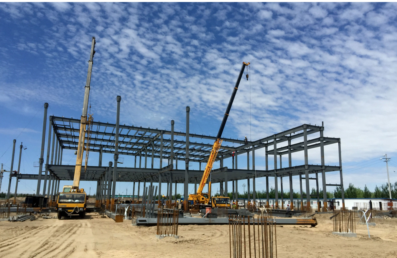
Phase I project of the Alibaba Cloud Zhangbei Data Center under construction in early of June, 2015 (Source: Qu Haifeng)
