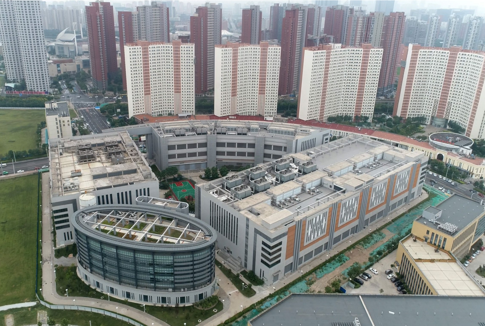
The Tencent Tianjin Data Center Campus is surrounded by the high-rise buildings. The chilled-water storage tanks are located close to Building 1, between Building 1 and 2. Building 3 has the largest capacity, which is about the sum of Building 1 and 4
