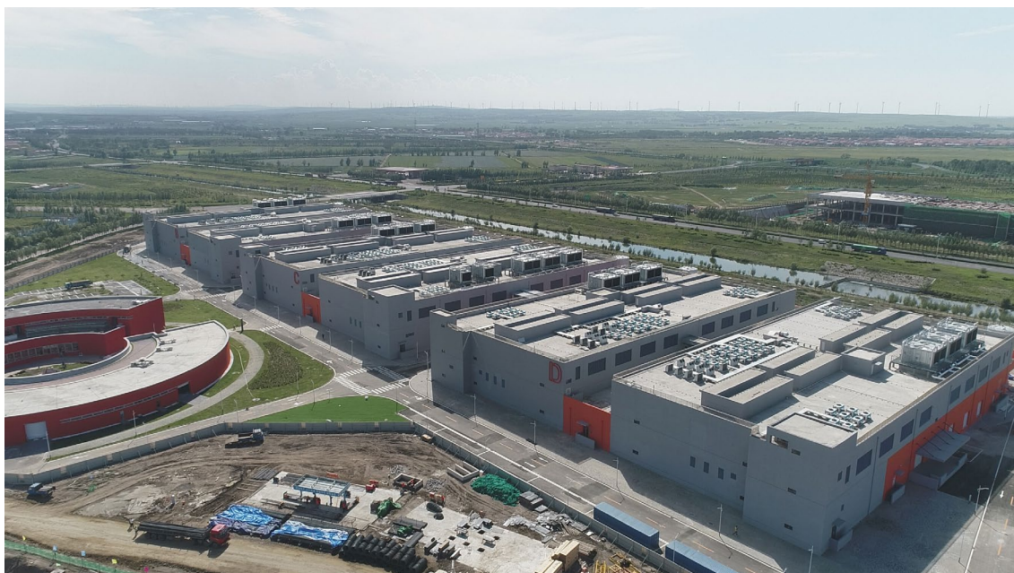
The wind power plants spread all over the No.1 and No.2 Campus of the Alibaba Cloud Zhangbei Data Center from a distant view
