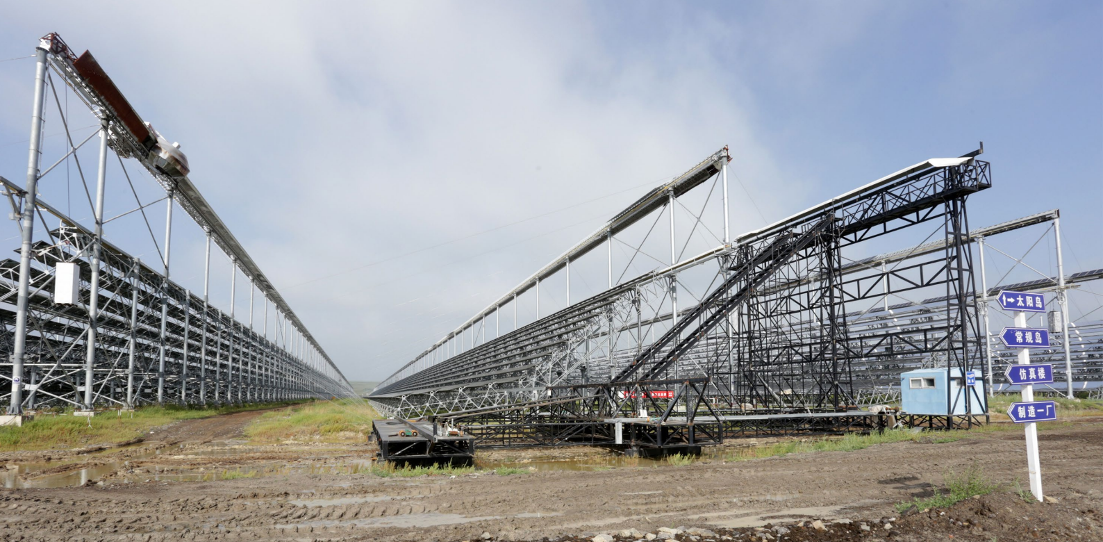
The North Mirror Field equipped with the Fresnel-like condensing mirror is called the "Sun Island", and the South Mirror Field equipped with the tower-type condensing system is called the "Conventional Island"
