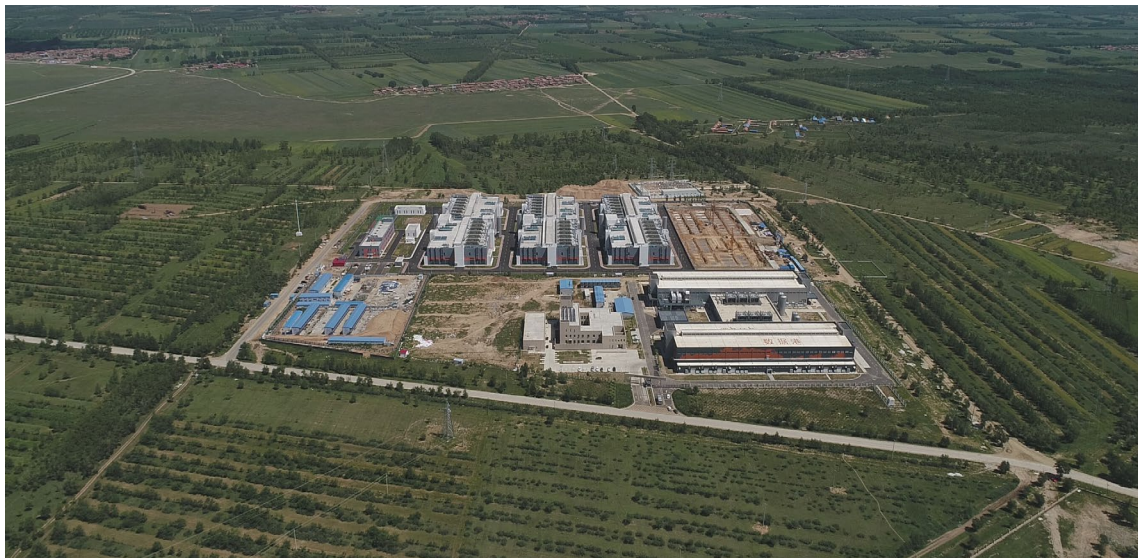
No.2 Campus of Alibaba Cloud Zhangbei Data Center under construction, the remote side is the substation of the Campus (August 10, 2018)
