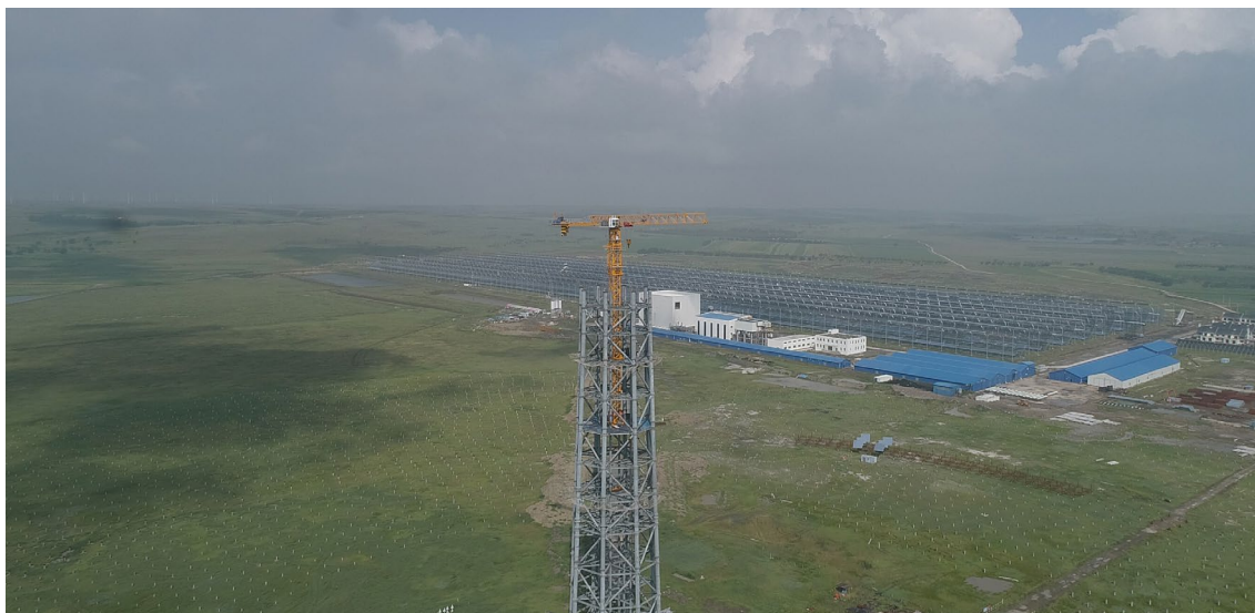
The South Mirror Field under construction and the North Mirror Field in the distance (the white cube shaped building is the thermal energy storage tower of the North Mirror Field) (at an altitude of about 1,500m)
