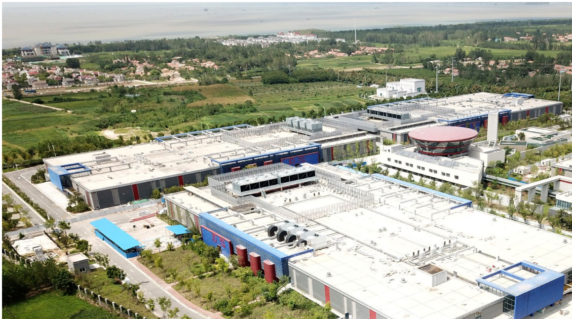
Partial of No.1 Campus in JD Cloud East China Data Center, the four equipment in the lower part of the central location are indirect evaporative cooling modules. The above plot across the road is planned to be the No.2 Campus, and the white building at the upper right is the dedicated 110KV substation
