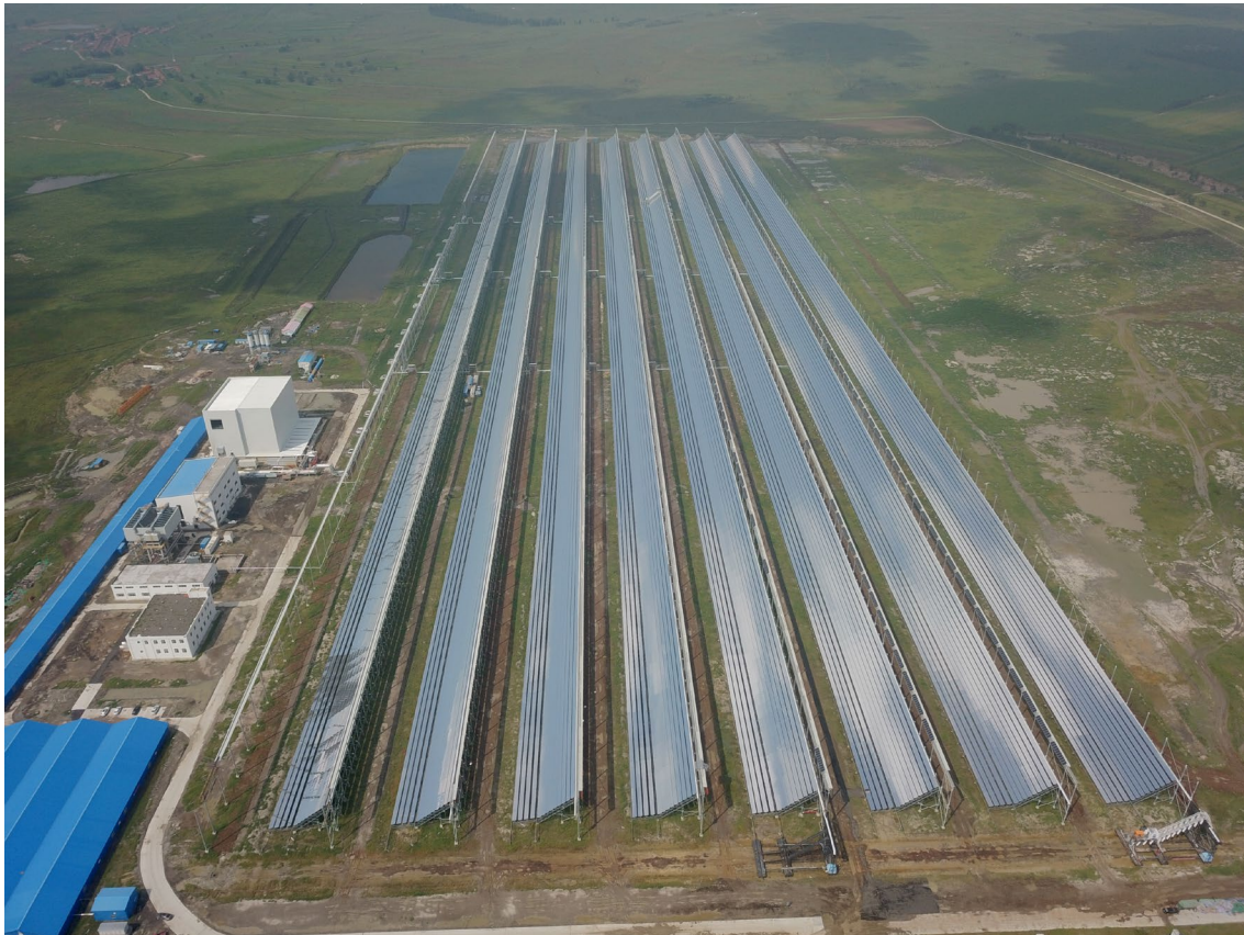
The North Mirror Field looks spectacular if you watch it standing on the roof of the building next to thermal energy storage tower on the left. Each of the specular arrays is more than 1km wide visually. There can have over 6,000 photovoltaic panels additionally installed to fully utilize the space on the top of the only 8 rows of arrays
