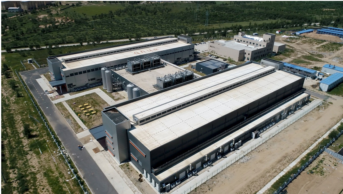
The Alibaba Cloud Zhangbei Data Center No.2 Campus - Phase I Project: it consists of two computer room buildings with the structural features of the chicken coop, which are connected by a cooling station in the middle; pay attention to the four chilled-water storage tanks on the side of the cooling station
