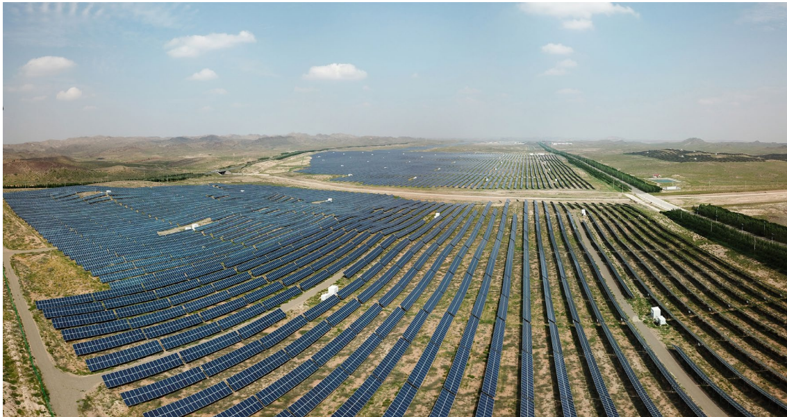
A PV power plant in the Zhongguancun Science and Technology Park - West Cloud Valley (altitude about 1,300m) in Zhongwei City, Ningxia Hui Autonomous Region; the data center and reserved land are in the distance
