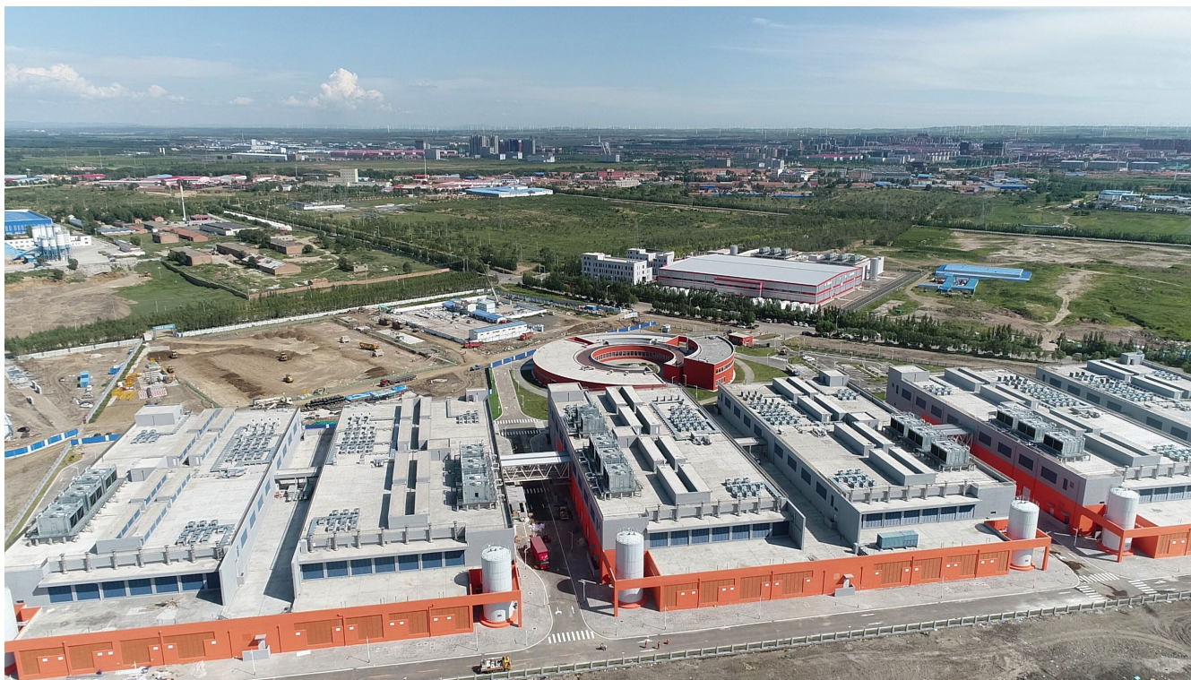
The Alibaba Cloud Zhangbei Data Center No.1 Campus - Phase II Project reflects the chicken coop style of the buildings, the fresh air cooling and direct evaporative cooling features, and the water-side free cooling features such as cooling tower and chilled-water storage tanks. All is for one purpose: making full use of natural cooling resources to save the operating expense (OpEx) even if the capital expenditure (CapEx) is increased
