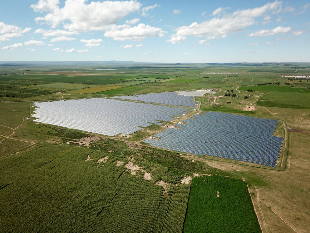
A PV power plant in Chahar Right Middle Banner region, Ulanqab City, Inner Mongolia, about 65km northwest of the urban area, altitude about 1,600m
