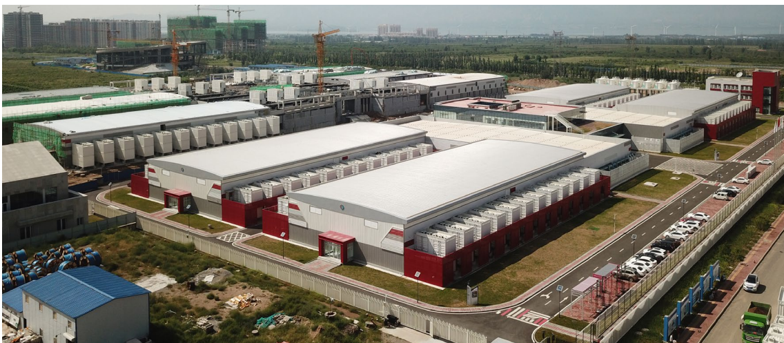
ByteDance Huailai Data Center on the afternoon of August 8, 2018: the completed 工 ("Gong", a Chinese character)-shaped building is Phase I Project, with a total of 4 computer room modules; Phase II Project (under construction, partially completed) is 王 ("Wang", a Chinese character)-shaped, with six computer room modules. Their middle part is the mechanical and electrical and office area, and the equipment similar to the container which are half surrounded by the red wall and are on both sides of the computer room modules are indirect evaporative cooling modules
