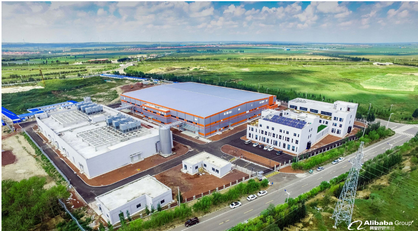
In the Phases I Project of the No.1 Campus in Alibaba Cloud Zhangbei Data Center, the white cooling station named as "Tianchi" connects to the two-storey computer room building through overhead water pipes. The plot at upper right across the road is that for the Phases II and III Project (not yet commenced in 2016)
