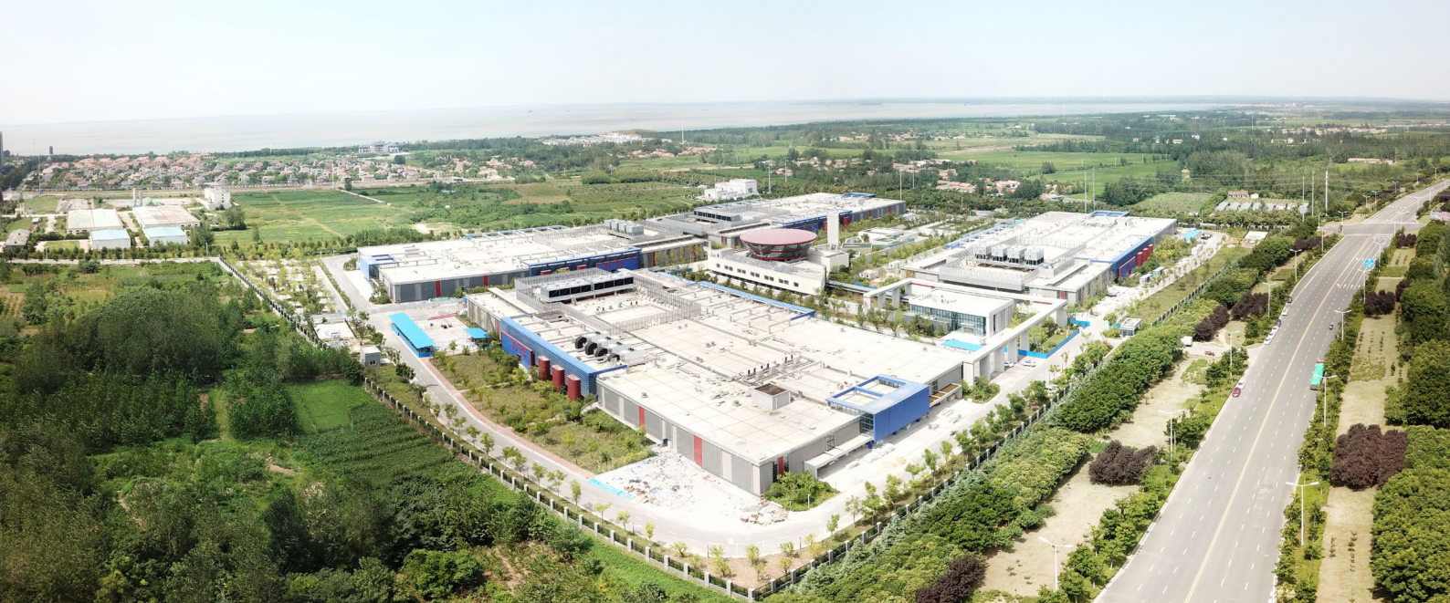
Panoramic view of JD Cloud East China Data Center, with the 4 computer room buildings in No.1 Campus completed and delivered in phases
