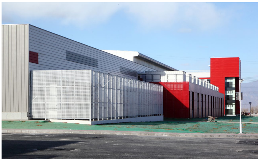
The white container-like equipment half surrounded by the red enclosure on the right side is the indirect evaporative cooling module for cooling the computer room. Those in the white enclosure on the left side are the equipment for cooling the mechanical and electrical modules and the equipment is replaced by the indirect evaporative cooling module installed on the top of mechanical and electrical modules area in Phase II Project
