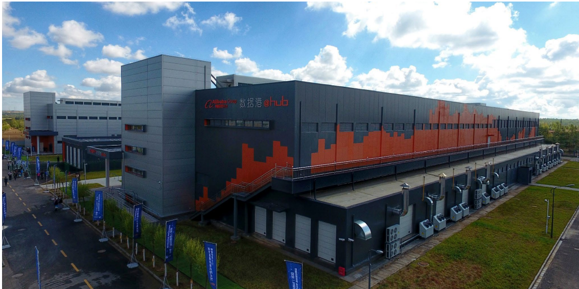
Phase I Project of No.2 Campus in Alibaba Cloud Zhangbei Data Center, where 8 diesel generators are put at one side of the computer room building, and the roller shutter door for the air intake and exhaust pipes can be seen from this perspective
