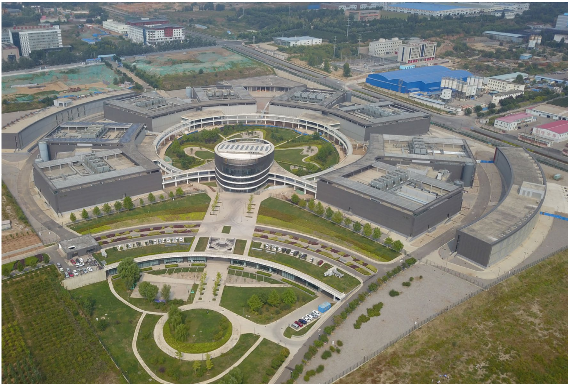
Baidu Cloud Computing (Yangquan) Center looks like a glowing light bulb, and it is inspired by the bear's paw of Baidu Logo. You can roughly see the chilled-water storage tanks placed next to the building and a variety of cooling equipment on the roof, mainly cooling towers, as well as indirect evaporative cooling modules. There is even a module that has solar panel installed on the roof
